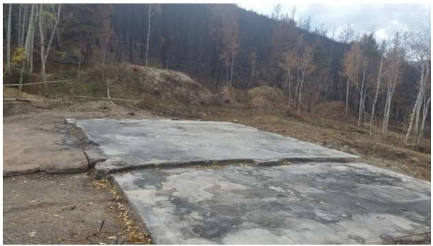
*Figure 3.* Foundation of an out building, located approximately 315 feet to the southwest of the main structures and 70 feet to the northeast of crown scorched trees, destroyed as a result of suspected ember ignition.
