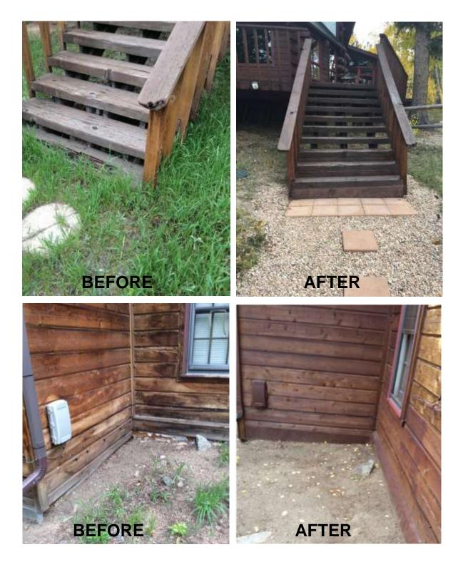
**Figure 1.** Before/After Mitigation Photos at 141 Sherwood Road (primary structure). Top left: condition of stairs and grass before mitigation (2014); top right: installation of a non-combustible border, repaired and sealed deck boards to eliminate any significant gaps or cracks (2016); bottom left: base of walls without flashing and vegetation (2014); bottom right: non-combustible metal flashing extending several inches from wall base, removal of all vegetation near structure (2016).
